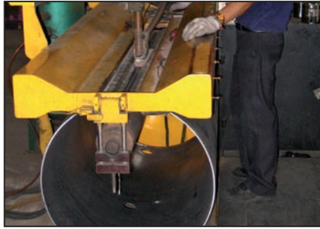
Longitudinal Joint Welding
